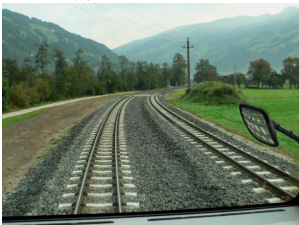
Selective upgrading of line by a second track Photo: Otfried Knoll
