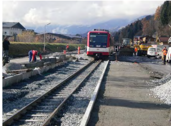
Reconstruction works Station Mittersill Photo: Ernst Lung
