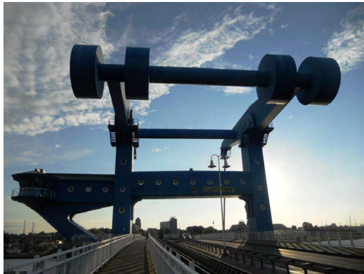
Combined bascule bridge for rail and road in Wolgast, photo: Otfried Knoll
