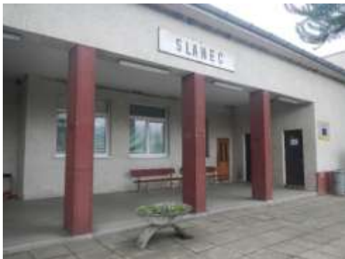
Railway station Slanec
